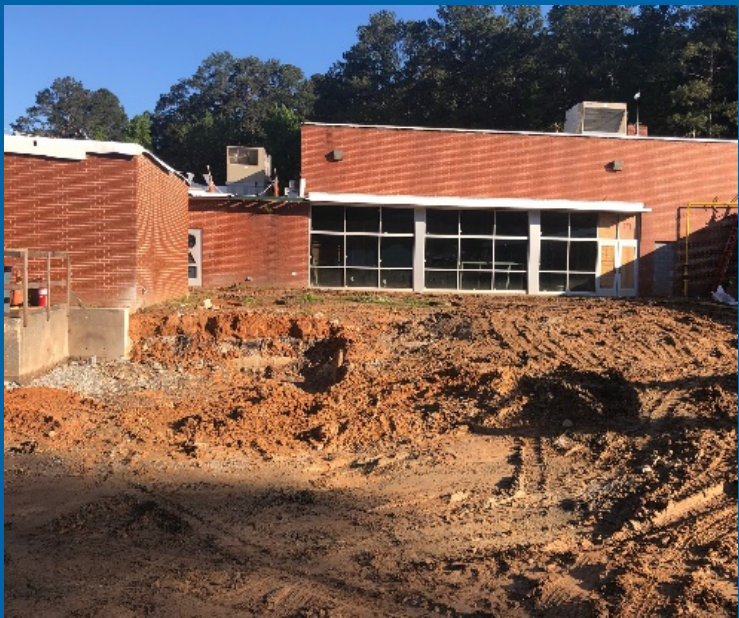
Site Demo Complete – Grading and Concrete to Follow
